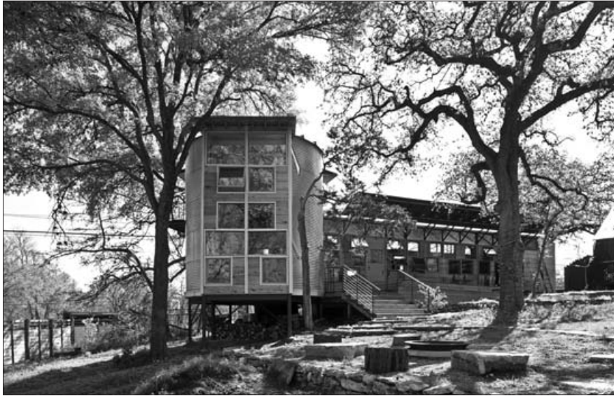
EM Franklin: 5 Etoiles. Photo : Kimberly Davis/Crédit Austin Energy Green Building Rating
